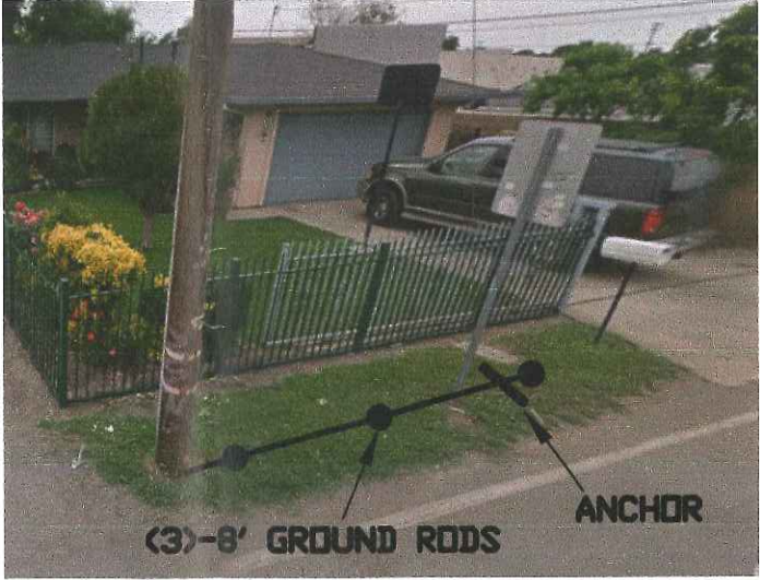
P.5A WORK AREA FACING WEST.
