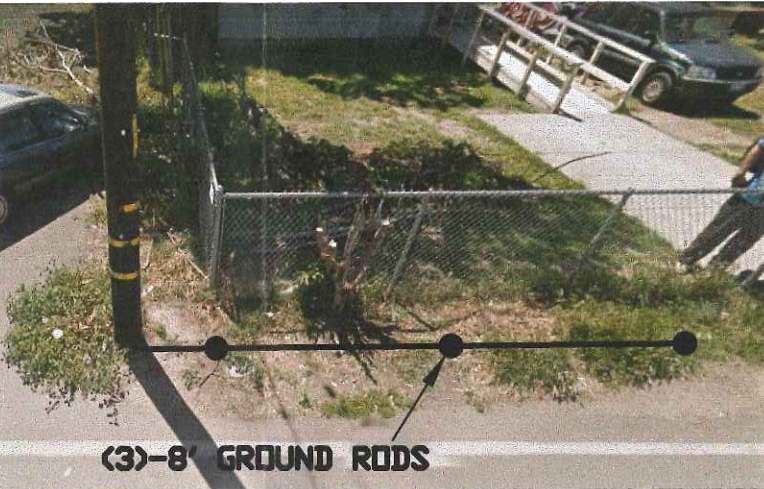
P.10 WORK AREA FACING WEST.
